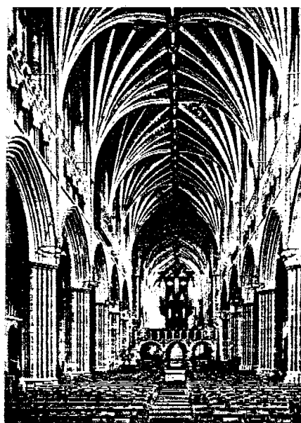
8. Rib vaulting in the nave of Exter Cathedral.
